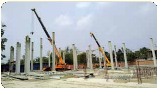
Steel Frame work
