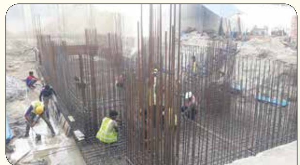
Rebar Fabrication
