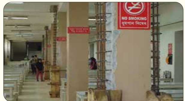
Retrofitted column at factory building
