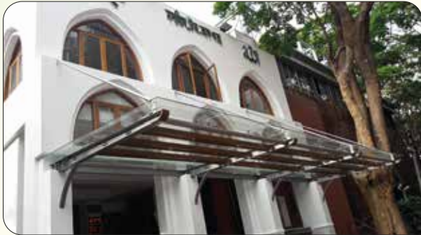
Canopy work: MASJID-UT-TAQWA
