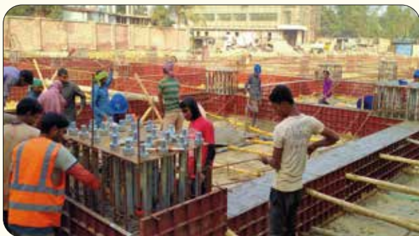
Anchor bolts fabrication for shed building
